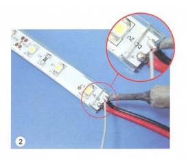
2. Rejoin the cables to the strip by soldering, please do not reverse the polarity.
